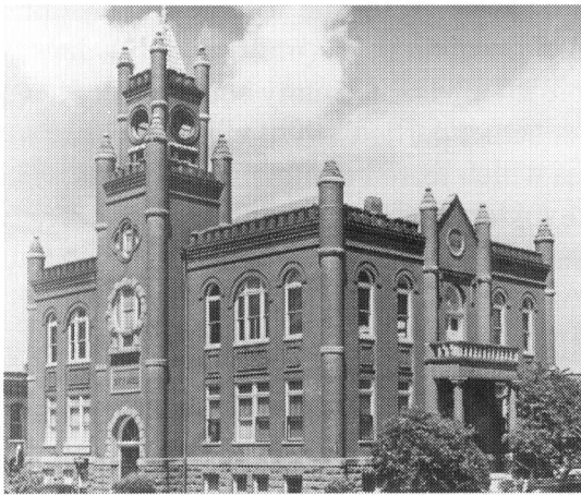
City Hall in Guthrie where the First Legislature met, 1907-8. Source: Bozarth Photography, Guthrie
