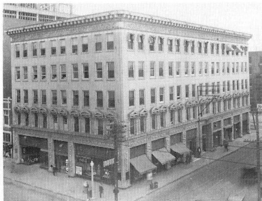
The Levy Building, later known as the Mercantile Building, where the Legislature met in Oklahoma City for 1910 Special and 1911 Regular Session. Source: Oklahoma Historical Society
